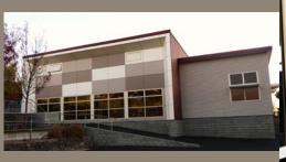
The design lent itself to creating enhanced visual appeal, especially on the West and South sides. A checkerboard effect with negative detailing was created where initially the full glass wall had been, allowing the front of the building to be determined. This was repeated on the West side in a simpler version. To add flow the checkerboard effect was repeated inside the building providing continuity.
