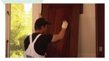
Once complete, wipe the door to remove the excess stain and to ensure an even coverage of the stain is achieved.
