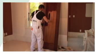
Start from the top and work down, working quickly to get the stain on the surface, laying-off with the brush as shown as you progress down the door.
