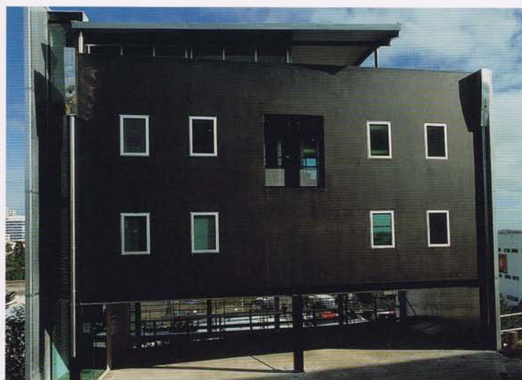
View of the Crosson office building from Augustus Street.
