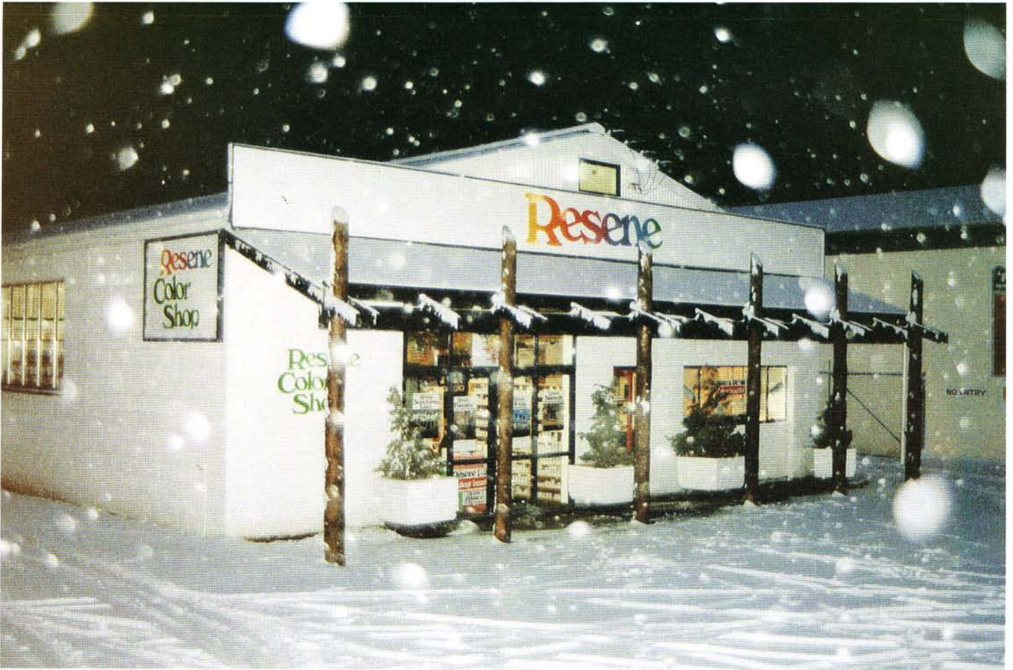
Snow falls on the new Resene Paints Color Shop, Queenstown.
