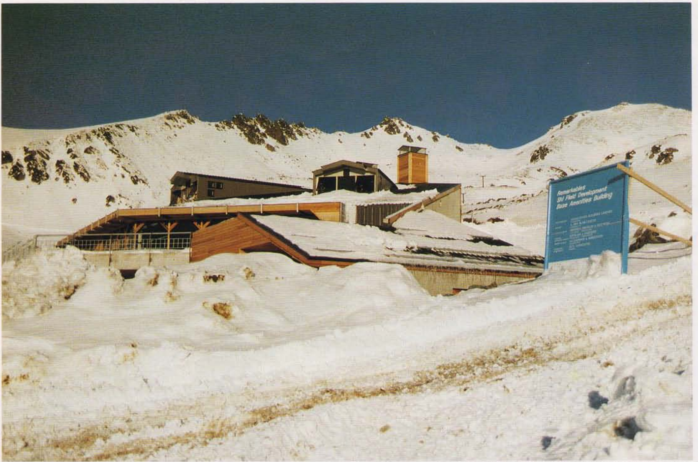
One of the many tourist and recreational developments being served from the new Resene Color Shop, Queenstown was the Remarkables Ski Field Base Amenities Building painted by John Henderson Ltd
