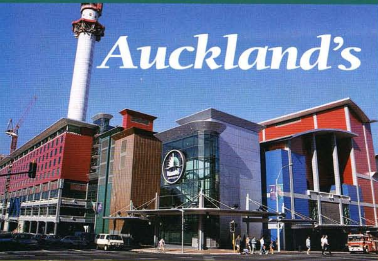
▲ An adhesion primer, Smooth Surface Sealer, was used in lieu of one of the coats of acrylic on the casino's pre-cast concrete exterior panels.
