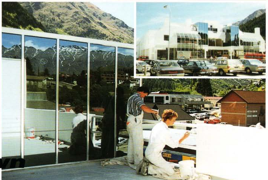
Paul Drysdale and Grant Smith finishing off the O'Connell Centre.
