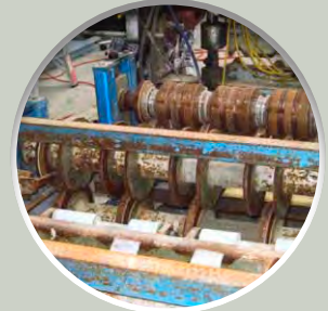
Laden with rust
