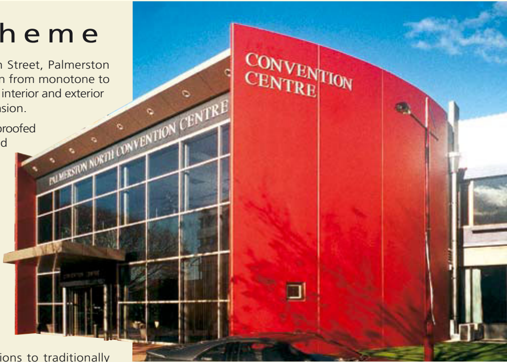
Architect: David Chapple, Susie Elms, Ian Clapham, Chapple Architects Painting Contractor: Tony Wright, Doug Miller Ltd Building Contractor: McMillan & Lockwood Palmerston North Resene: Dave Sargent, Manawatu Branch Manager
