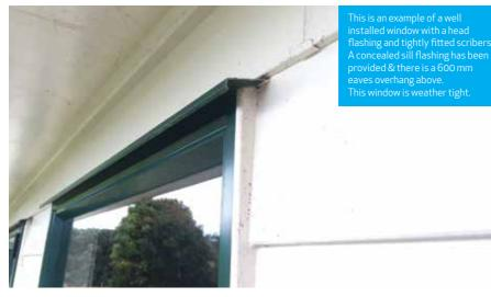
"A lot of weatherboard houses built in the 1980s and 1990s didn't have scribers – a vertical timber board that runs along the side of the window and fits tightly into the cladding. That caused a problem. A scriber can be easily fitted by someone with basic handyman skills. Check Google or Youtube for instructions.
