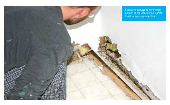
Houses with masonry perimeter foundations tend to lack ventilation. Or homes where fibrolite or cement fibre have been used as a sub-floor cladding. "You need a good amount of ventilation around the sub-floor so air can flow from all four sides. Sometimes you don't get that. If it's vented on one side, it won't vent well. I often see fungus growth on the ground here. Or particle board flooring becomes damp and fungus grows on the underside," Turner says.
