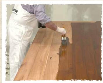
3. Wipe the surface using a clean lint-free cloth to remove excess stain and ensure the stain is evenly applied to the timber. Have additional cloths ready to replace saturated cloths as you progress. This is very important for large areas especially floors and sheets of plywood and MDF. Allow to dry.
