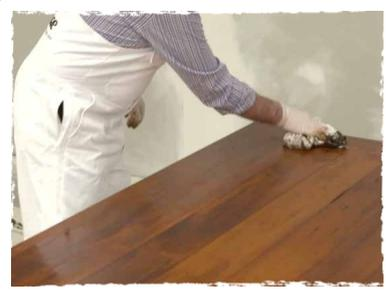
4. Apply Resene Aquaclear or Resene Qristal Clear polyurethane in your desired gloss level. For flooring apply Resene Qristal ClearFloor.
