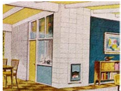
Interior concrete block walls and raised fireplaces.
