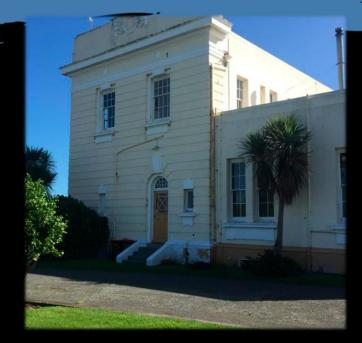
Paint coatings on North facing timber will have a far shorter expected life span than paint coatings on South facing concrete. Coatings on substrates that are affected by heat stress will have shorter lifespan than coatings on substrates that aren't
