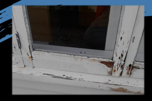
North facing timber joinery, particularly sills, is affected significantly more due to it's angle to the sun which increases UV impact
