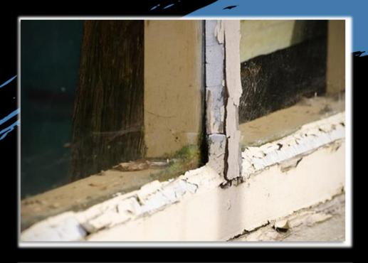
1. Water seeps into the crevice, cracks and between the glass/putty, which causes stress to be placed on and within the timber and paint film, splitting at any grain boundary weak point.
