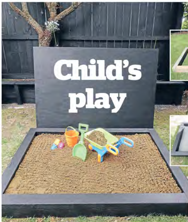
Put the timber framing together (using H5 1500x100mm pine in this case). Photos: Sarah Withell
