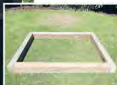
Put the timber framing together (using H5 1500x100mm pine in this case). Photos: Sarah Withell
