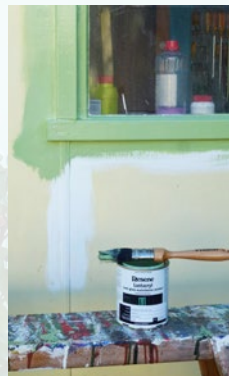
Step seven Apply two coats of Resene Woodstock to the window frame and surround, allowing two hours for each coat to dry.
