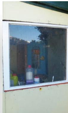
Step three Fit the wooden framed window into position, as shown.
