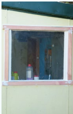
Step five Fill any gaps and seal around the window with flexible filler. Allow to cure.
