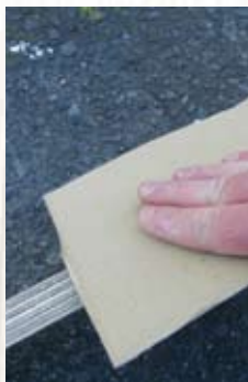
Step two Smooth any rough edges with sandpaper.
