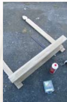
Step four Attach the lower shelf to two of the fence pickets, as shown, fixing with PVA glue and nails. Leave a gap of 30mm at the bottom edge and use a set square to check the pickets are at right angles.
