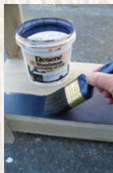
Step seven Apply two coats of Resene Woody Bay to the entire unit, allowing 24 hours for each coat to dry.
