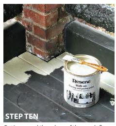
Cut in around the edges of the porch floor with Resene Walk-on flooring and paving paint.
