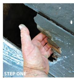
Carefully lift any rotten timber, as shown.
