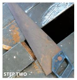
Mark and cut across the timber, removing the rotten section. Ensure the cut is halfway above a support joist.
