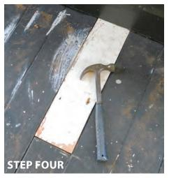
Fix the timber to the joists below using decking nails.
