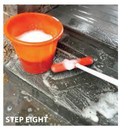
Scrub the solution vigorously into the porch flooring using a broom. Allow to remain wet for 15 minutes and then rinse thoroughly with clean water. Allow to dry.
