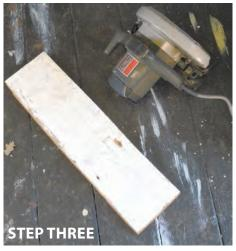
Measure, mark and cut a piece of timber to replace the rotten section.
