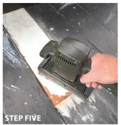
Fill the join and any other gaps in the existing timber with exterior filler and allow to dry. Sand the filled areas smooth.
