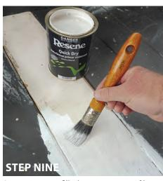
Spot prime any filled areas or areas of bare wood with one coat of Resene Quick Dry and allow two hours to dry.
