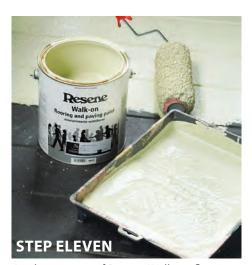
Apply one coat of Resene Walk-on flooring and paving paint to the rest of the porch floor. Allow to dry and then apply a second coat of Resene Walk-on flooring and paving paint. Allow to dry.
