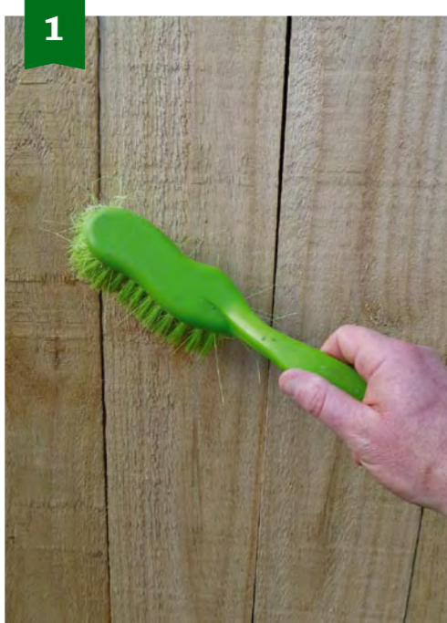
Remove any dust and dirt from the fence using the stiff-bristled brush.
