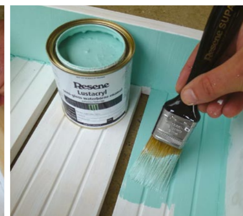
Step 9 Apply two coats of Resene Renew to the entire box, allowing two hours for each coat to dry.
