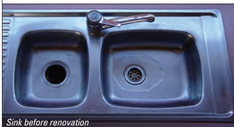
Sink before renovation
