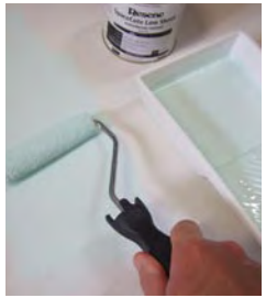
Step one Apply one coat of Resene Quick Dry to the MDF panel and allow one hour to dry.
