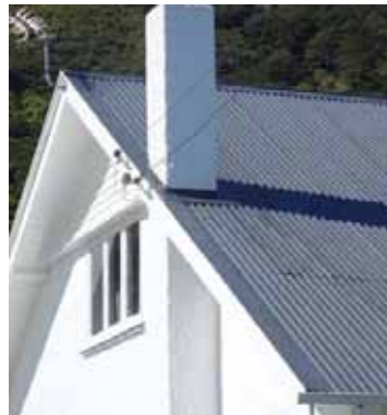
An example of corrugated iron roofing.
