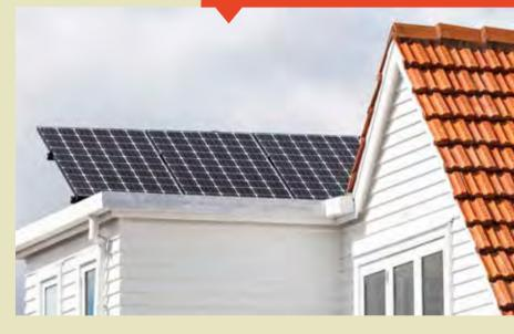
The average household uses about 22 kilowatt hours of electricity per day which requires about 45 square metres of PV panels on the roof. The average roof has much more area than that, so this is easily achievable.
