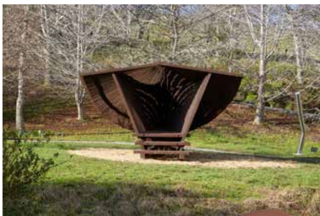
above: The Nest (top) currently sits in the same location as the previous folly from which its materials were extracted, The Wood Pavilion (bottom). Leo Zhu, Dorien Viliamu, Daniel Fennell and Wenhan Ji designed and built The Wood Pavilion in 2019 and stained it with Resene Woodsman Bark wood oil stain. The timber was upcycled to create The Nest and is painted in Resene Lumbersider Low Sheen tinted to Resene Toorak (outside), Resene Lone Ranger (inside) and Resene Okey Dokey (timber length ends).
